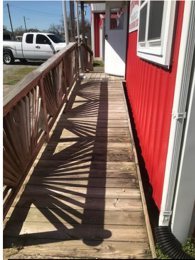
Non-Compliant Ramp at Main Entrance
