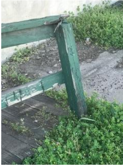
Damaged Guardrail on Ramp
