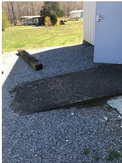
Non-Compliant Ramp on Side of Building
