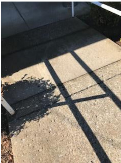
Crack in Surface of Ramp
