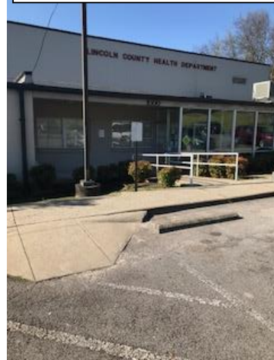
Unlevel Space, Improper Curb Ramp in Front Lot
