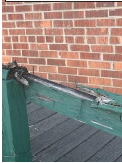
Damaged Handrail on Ramp
