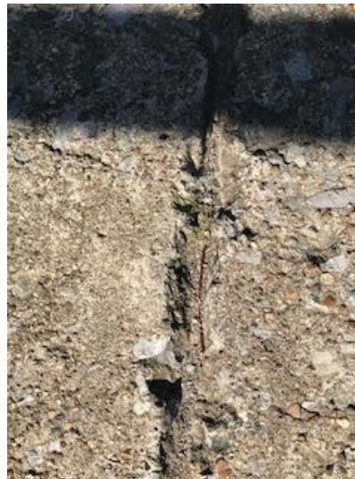
Detail of Crack in Ramp Surface
